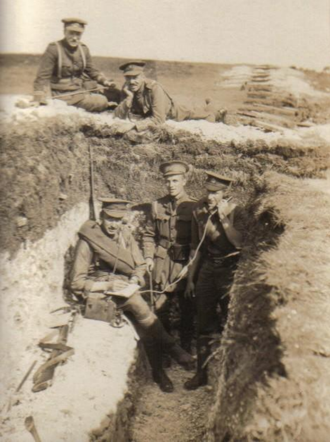
Telephone station, practice trenches, Barham, Kent.
