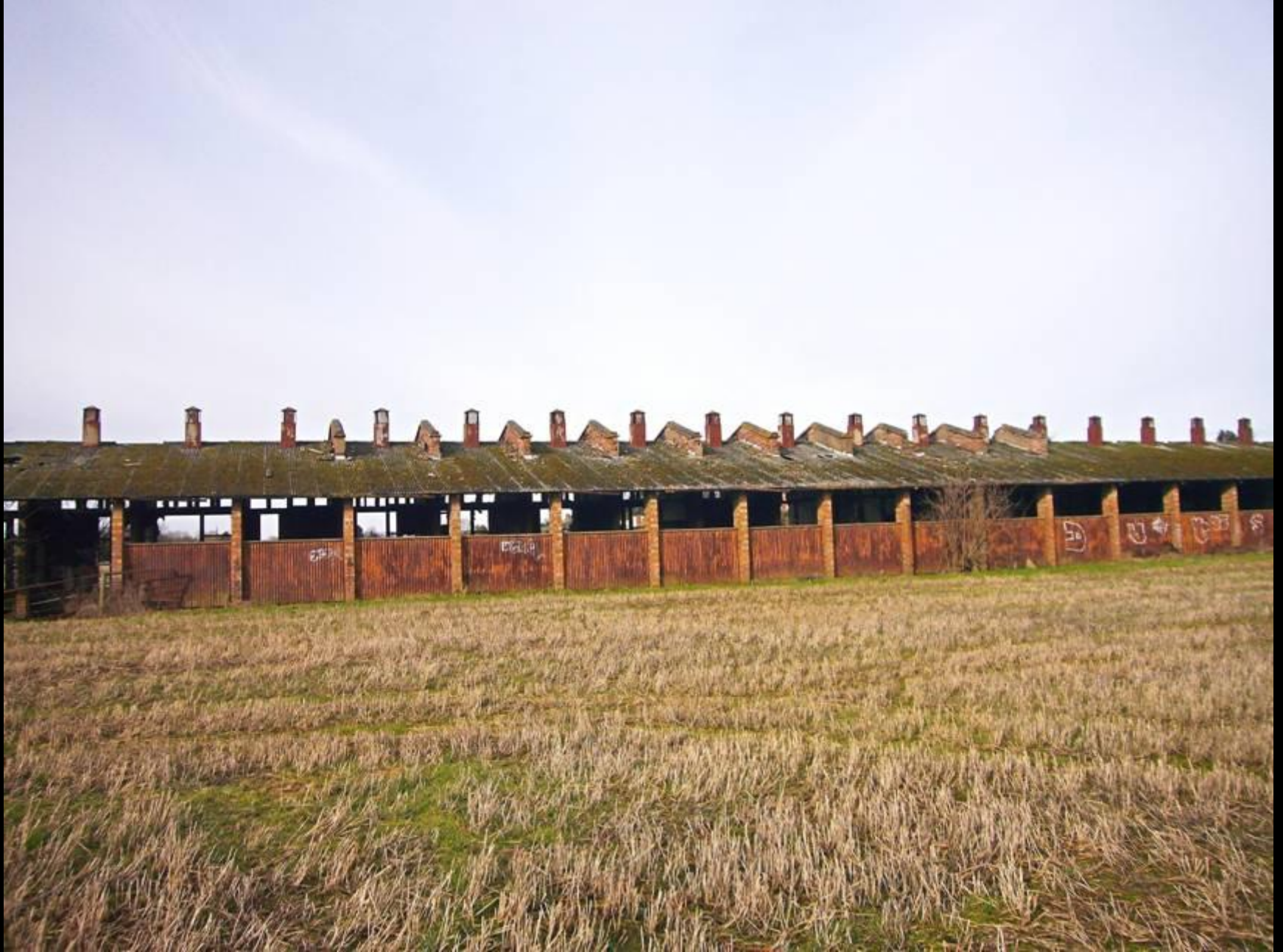
Rotherwas, Herefordshire: Picric Acid Store (listed Grade II)
