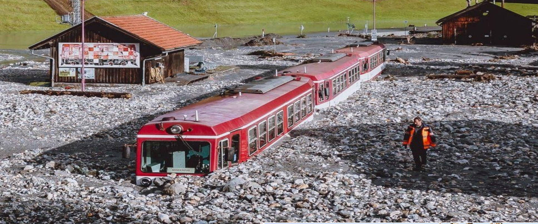
Austrian flood damage
