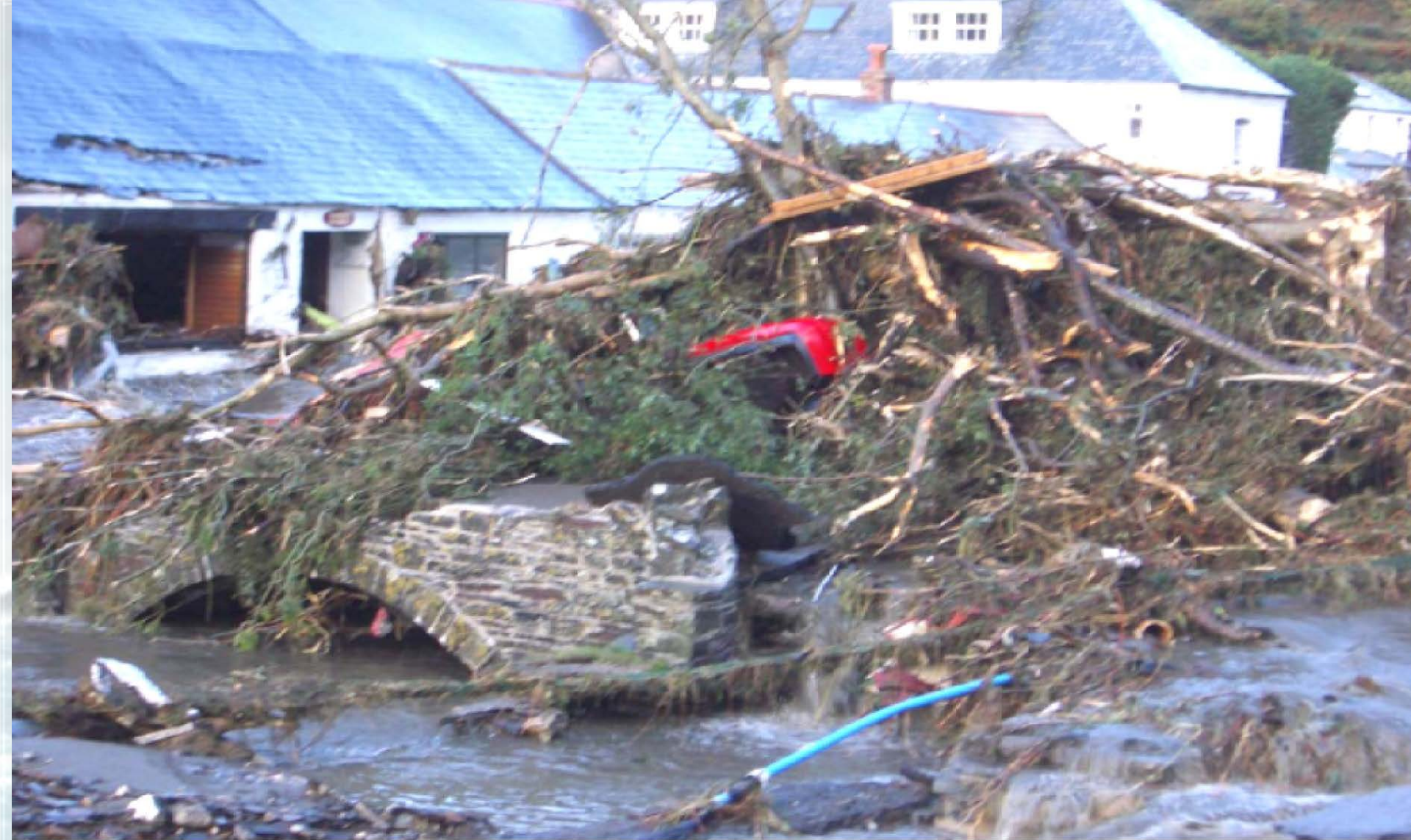
A bridge blocked by vehicles and debris during the 2004 Boscastle flood ( http://www.tintagelweb.co.uk ).
