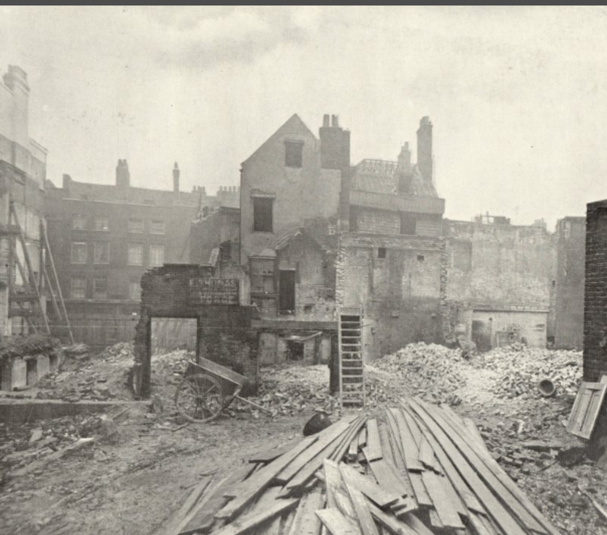
Little Wild Street in the course of demolition
