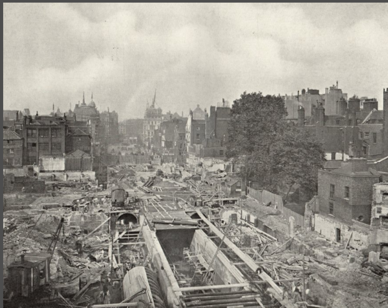
Excavations in Kingsway
